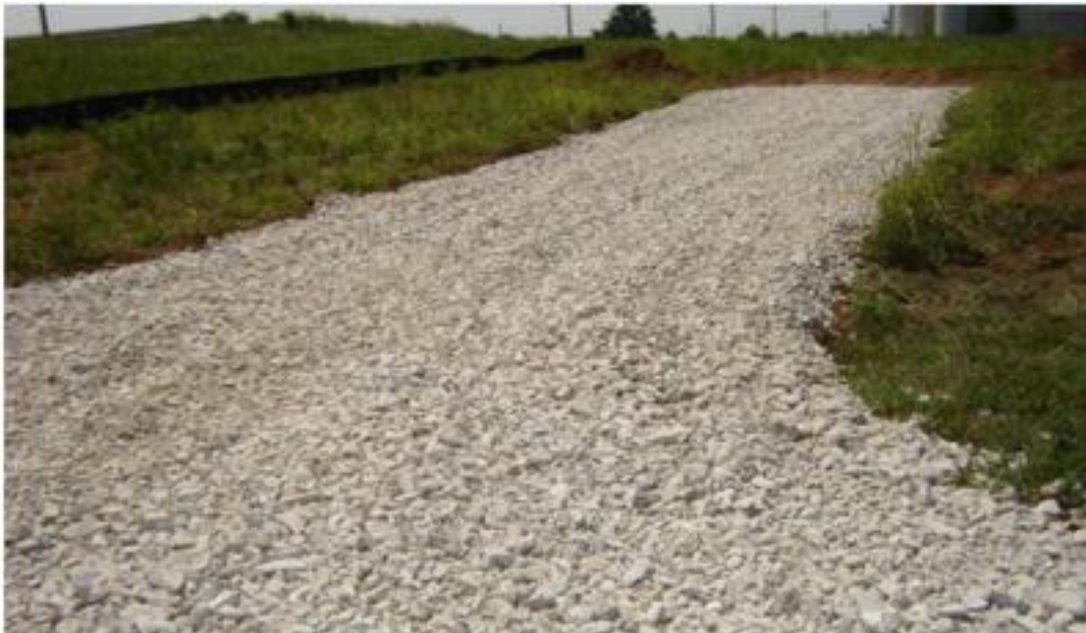
Plate 5: Temporary access track
